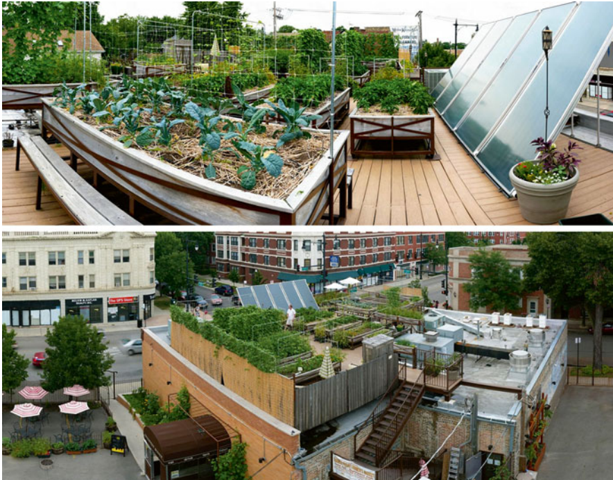
Fig. 7 Rooftop gardens at the Uncommon Ground restaurant in Chicago, IL (Photo by Zoran Orlic www.zoranorlic.com )
